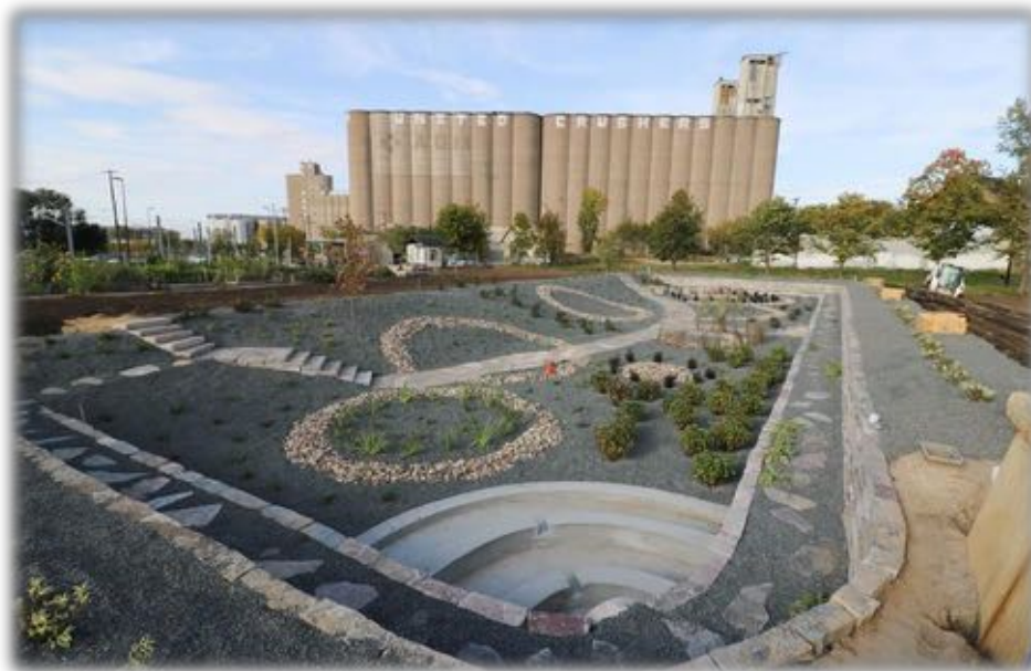
Figure 7. The gateway to Prospect North. ADM-Delmar #4 Elevator (1931), known as “United Crushers,” forms a prominent backdrop to community gardens and open space envisioned as a future urban park. In the foreground is an innovative district stormwater facility built through partnerships with MWMO and Towerside.
